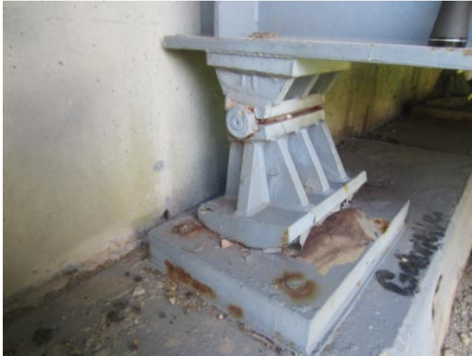
Left outside rocker over abutment #4
