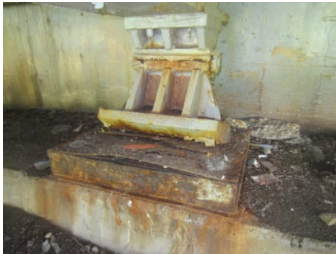
2nd rocker from left over abutment #1
