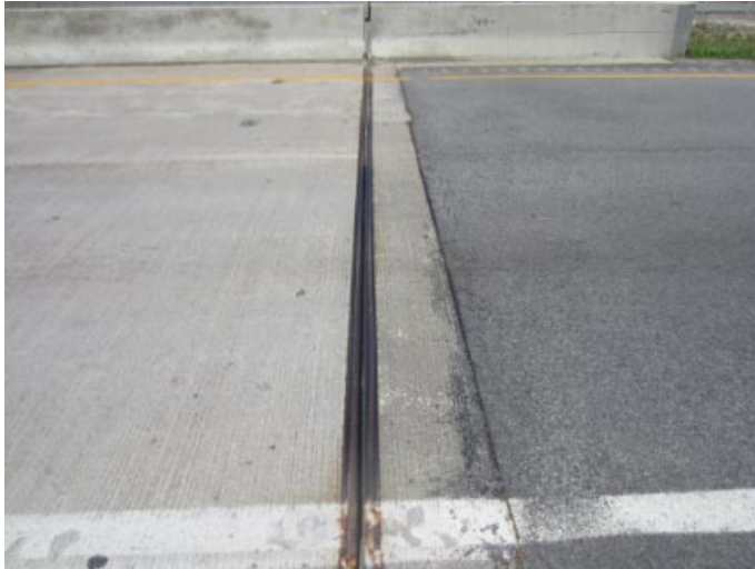
Looking left across strip seal expansion joint over abutment #4
