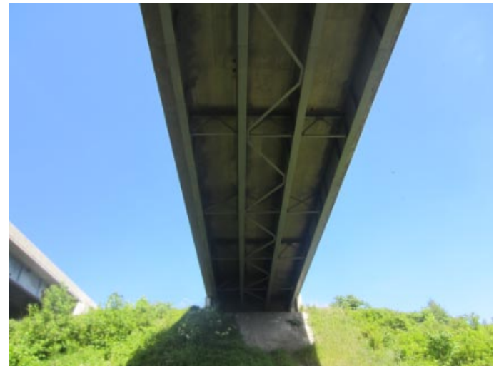
Looking east along bottom of superstructure in span #3
