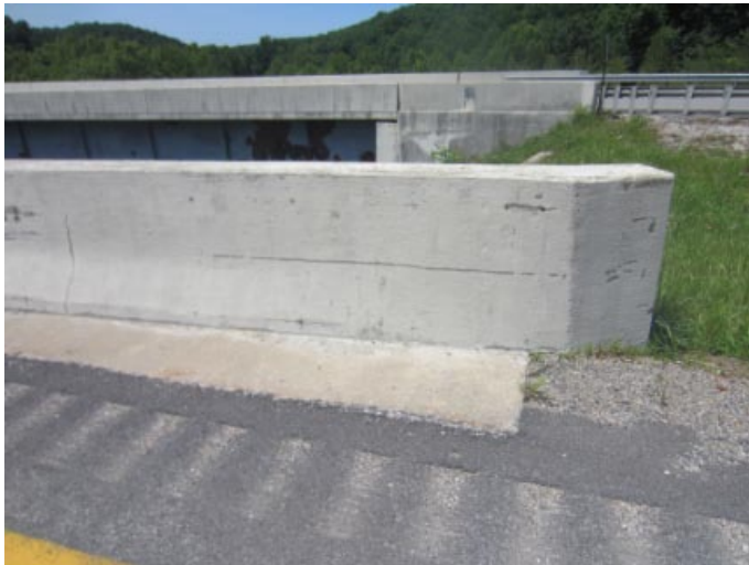
East end of left side parapet
