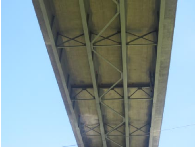
Looking east along bottom of center span
