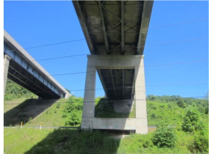
West face of #3 pier
