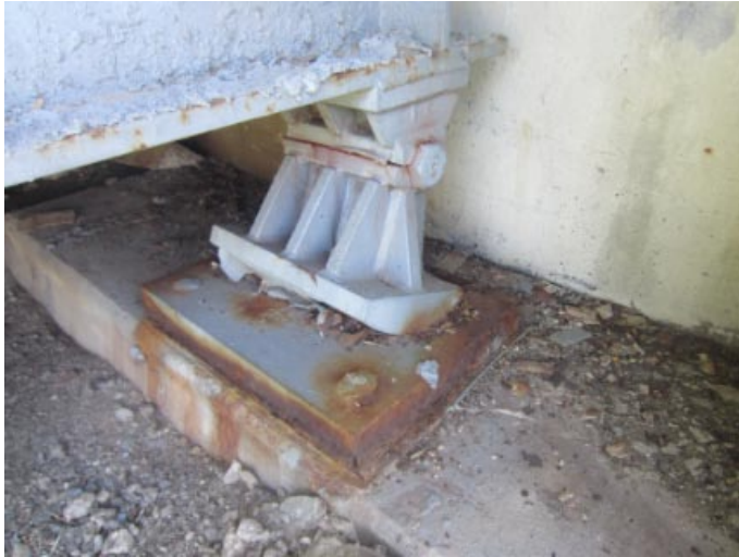
Left outside rocker over abutment #1
