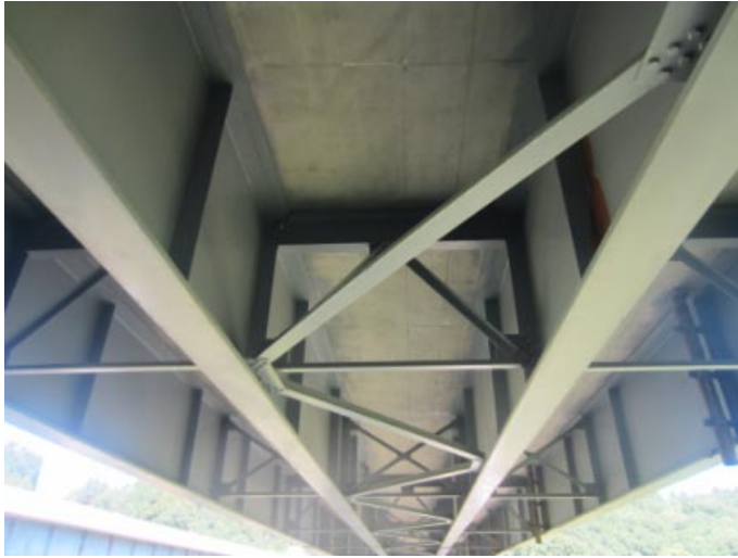
Looking east along span #1
