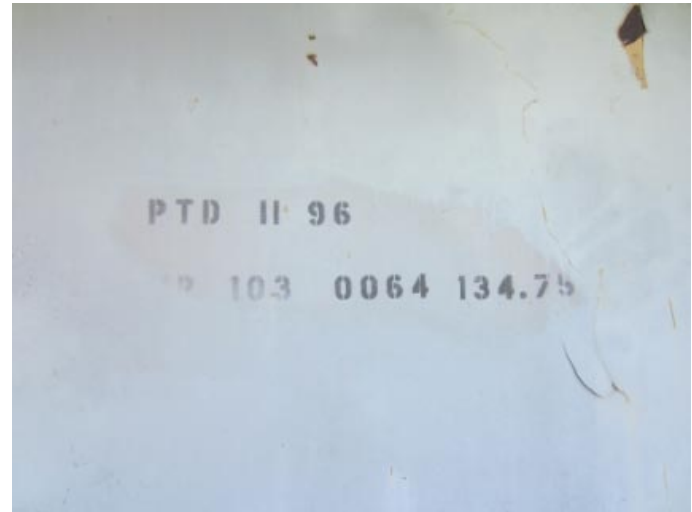
Paint information on left outside face of superstructure next to abutment #1
