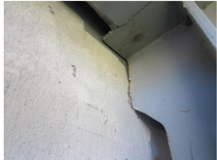
Left outside beam tight against abutment #4 backwall
