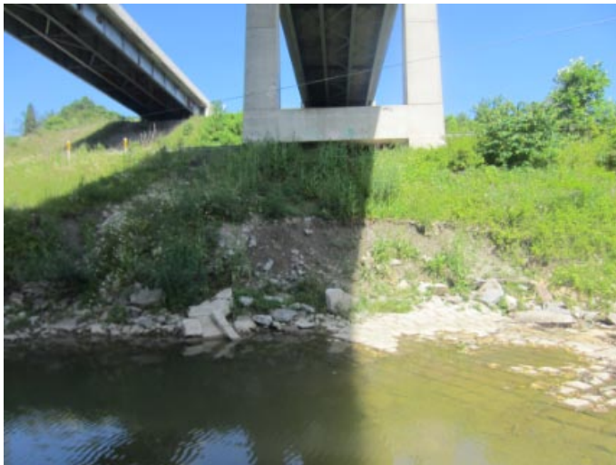
East stream bank under bridge in center span
