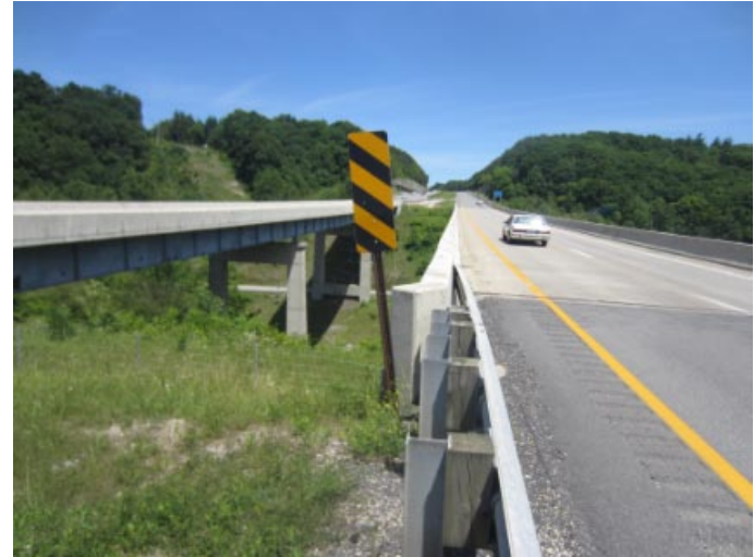
Left side obstruction marker at abutment #1
