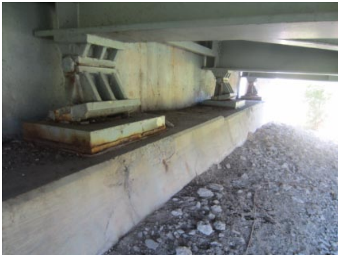
Looking right along abutment #4
