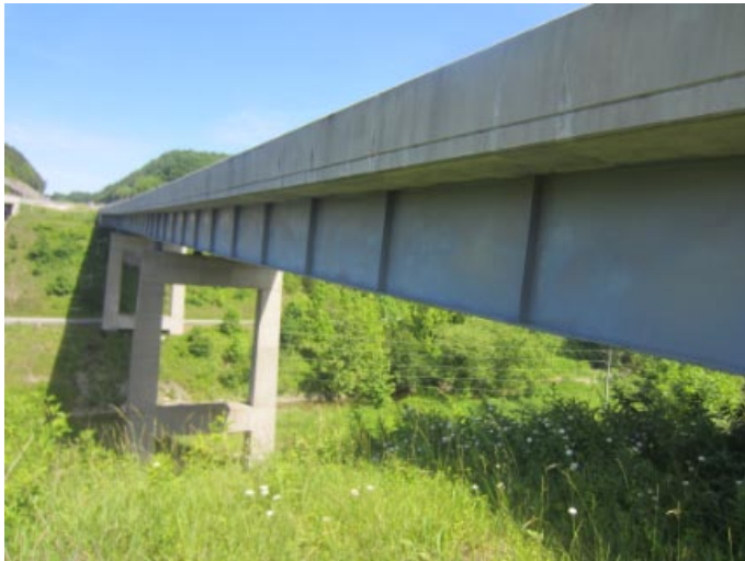
Looking east along left side of bridge
