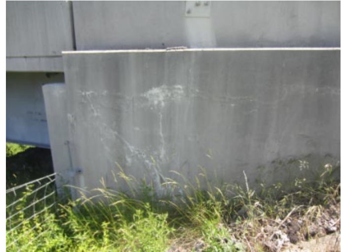
Left outer end of abutment #1
