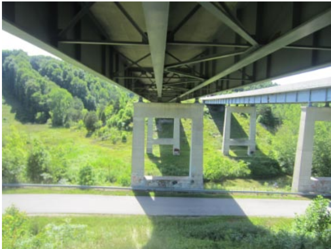
Looking west along bottom of span #3
