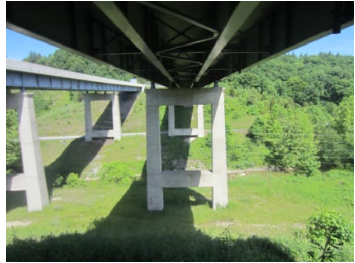
Pier #2 west face
