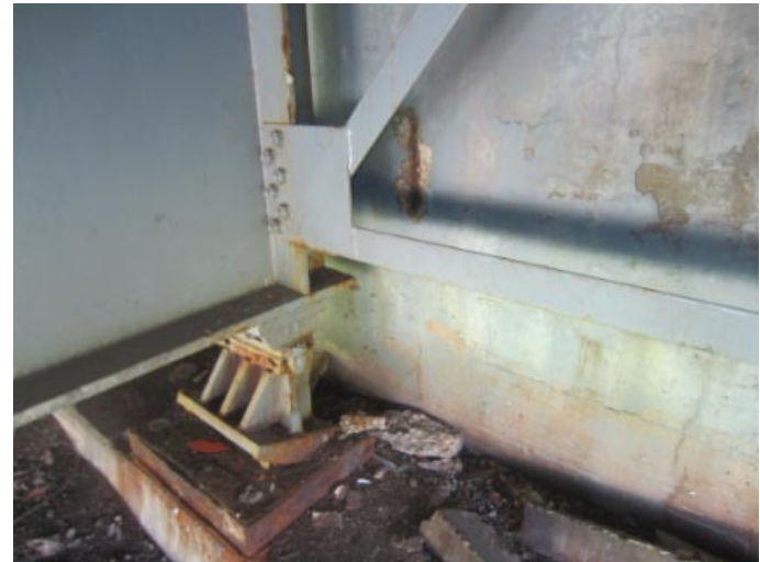
Abutment #1 at 2nd rocker from left
