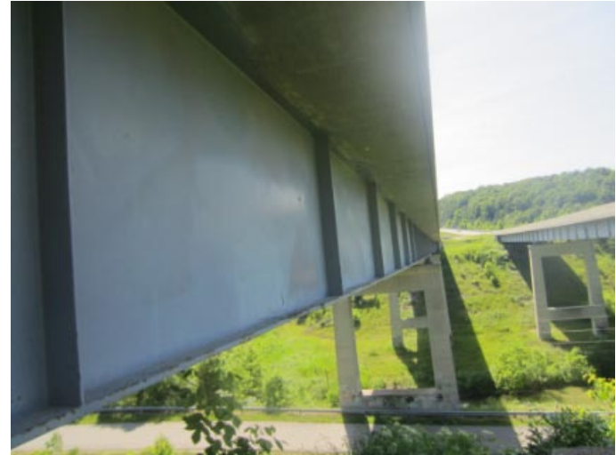
Looking back west along left face of superstructure
