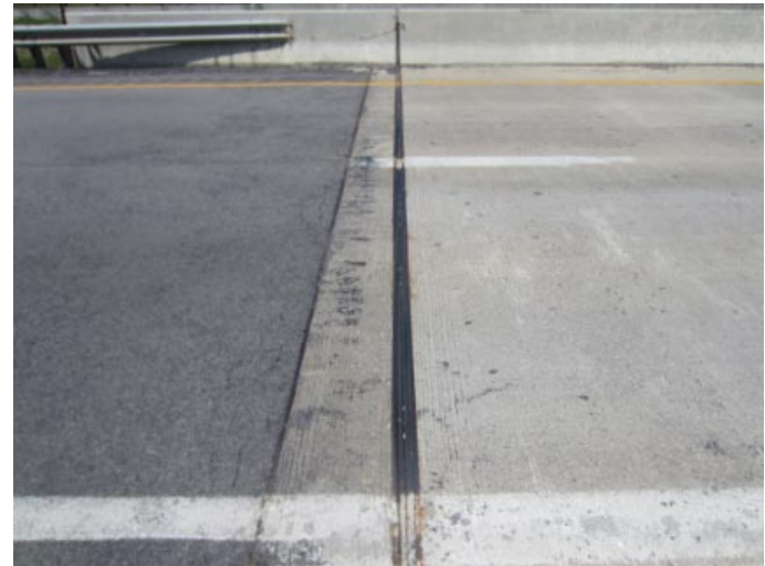
Looking left over compression seal expansion over abutment #1
