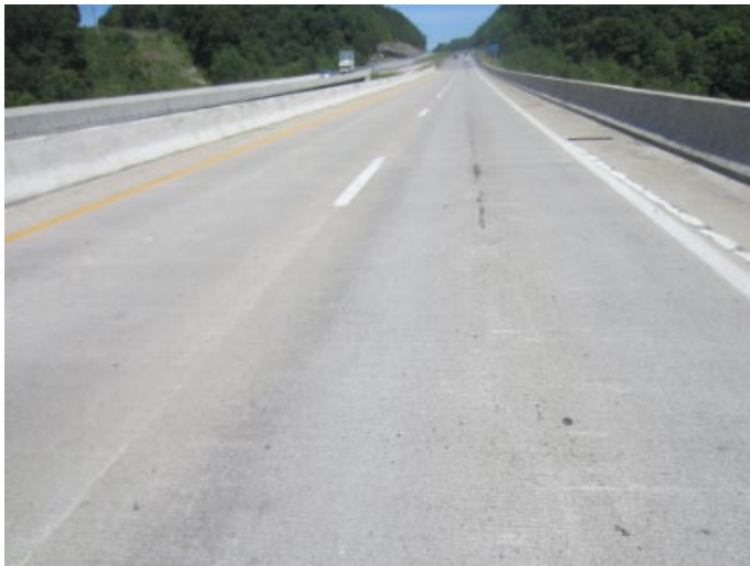
Looking east over main drive lane
