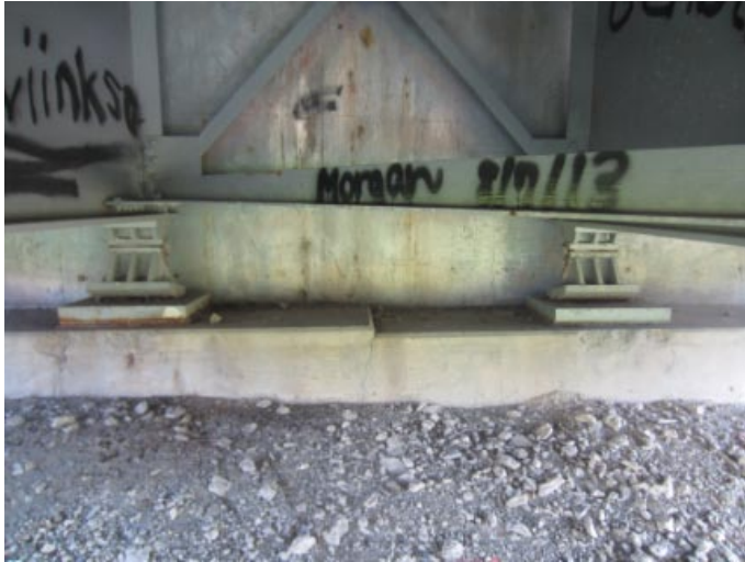
Center of abutment #4
