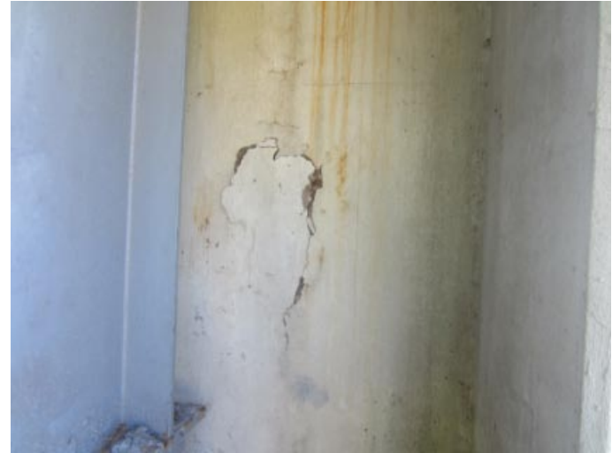
Abutment #1 backwall next to left end
