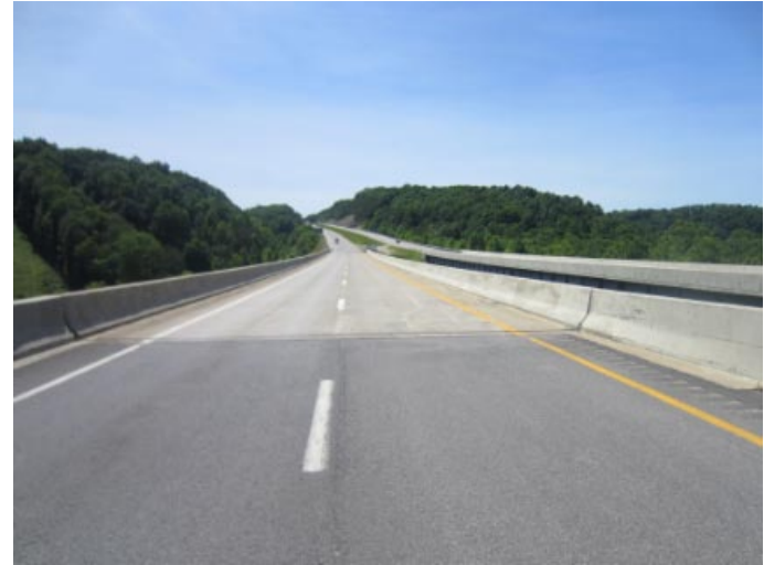
Looking west back over bridge
